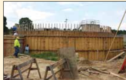
Construction of one additional aeration basin.
