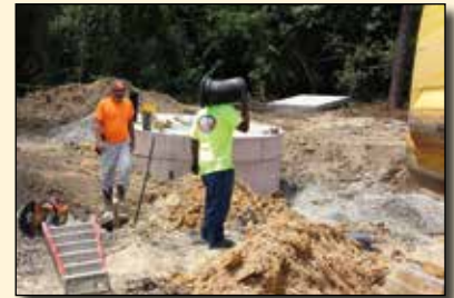
Crew members work on lift station number 2.
