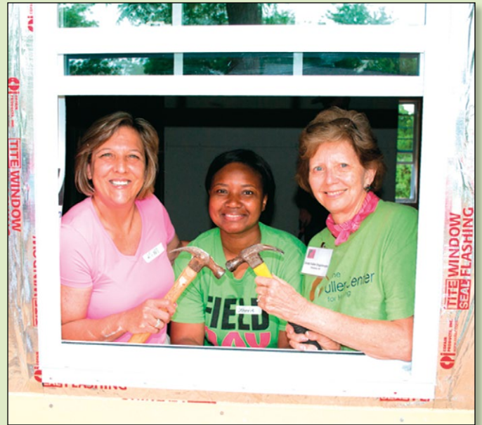
From left, Chattahoochee Fuller Center Project (CFCP) Executive Director Kim Roberts, new homeowner Jetorrie Johnson and Fuller Center for Housing Co-Founder Linda Fuller Degelmann celebrate the progress made in building CFCP Home No. 34 in Lanett this past June. This was the first home built by the Fuller Center with all of the work being done by women. (Photo by Wayne Clark)
