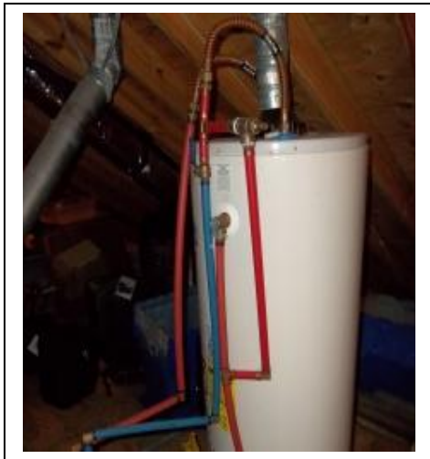
Retrofit Pressure Relief Valve for Water Heaters With added High Temp. Blow-off Valve
